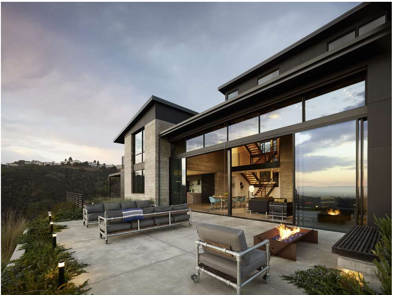
Rick Campi Construction worked with contractors to develop the incredible concrete floors and walls. Photos by Matthew Millman .
